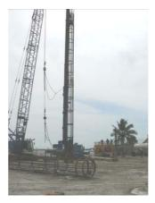
Multi-level O-cell cage ready for installation
